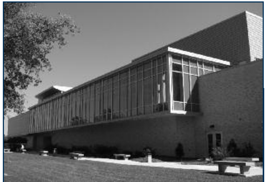
The new Health Sciences Library and Learning Center opened its doors in January 2007.
